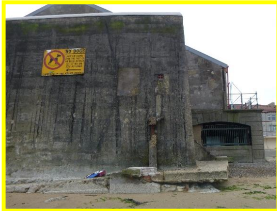
Cinema seawall (/C0602C05)
