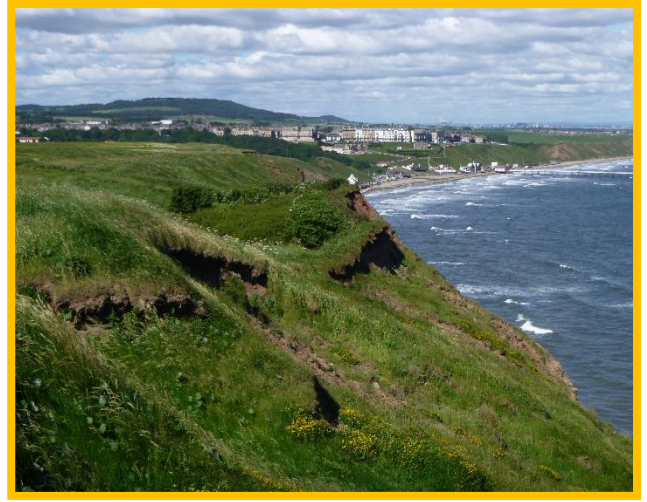
Suspected approximate location of rockfall E53/2 (Partly Active).
