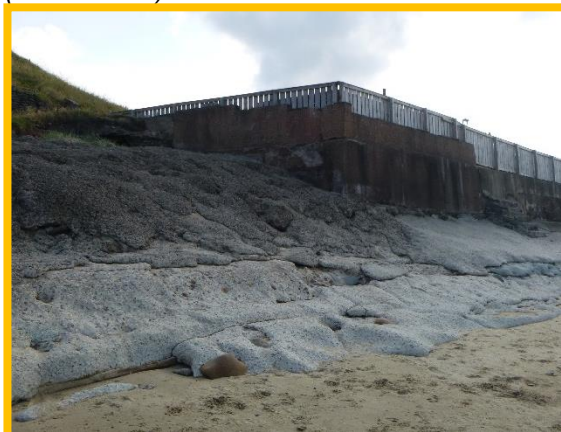
View looking west (/C0704C05)
