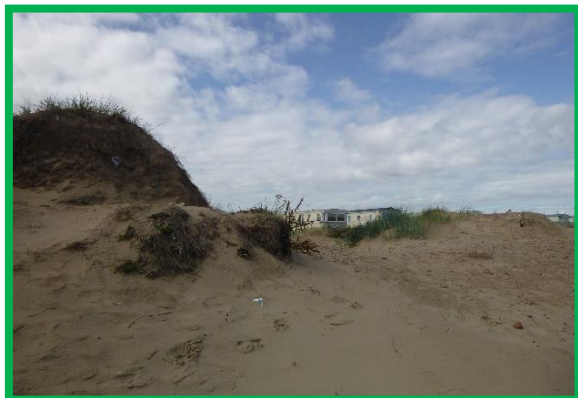
Loss of dune crest at access point (/C0507C01)
