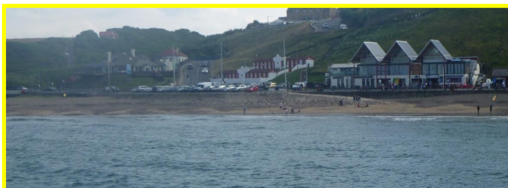
View looking southeast from pier. Beach levels lower at ‘apex’ of headland (/C0704C01)
