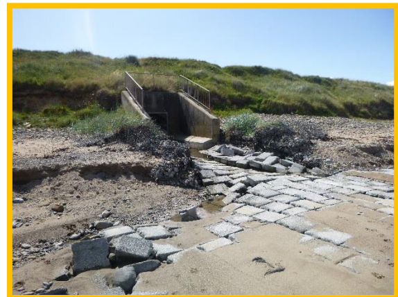
Concrete outfall structure (/C0701C01) CBU E52/10
