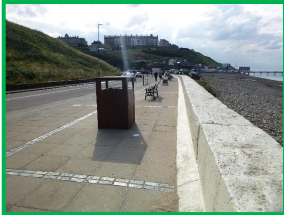
View looking west (/C0704C03)
