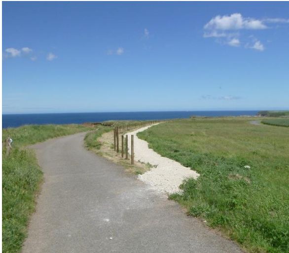
E59/4 work ongoing to further abandon a section of the old Cowbar Lane road, now access is restricted to users of the Cleveland Way path.
