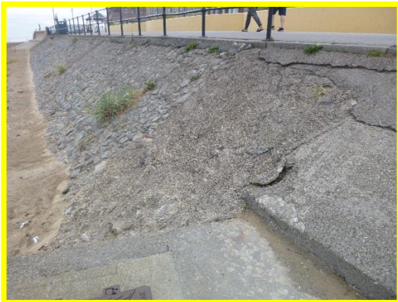
Grouted stone revetment (/C0601C01)
