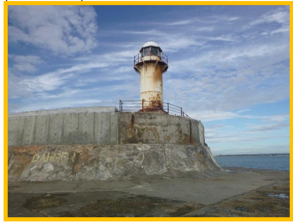
Northern extent of upper structure (/C0506C01)
