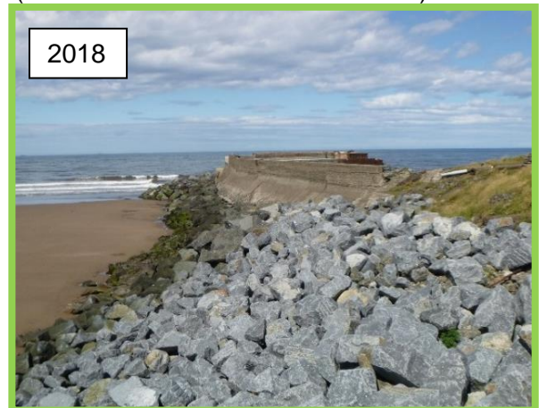
Repaired and improved rock armour (Asset Ref No. 1221D901D0201C02)
