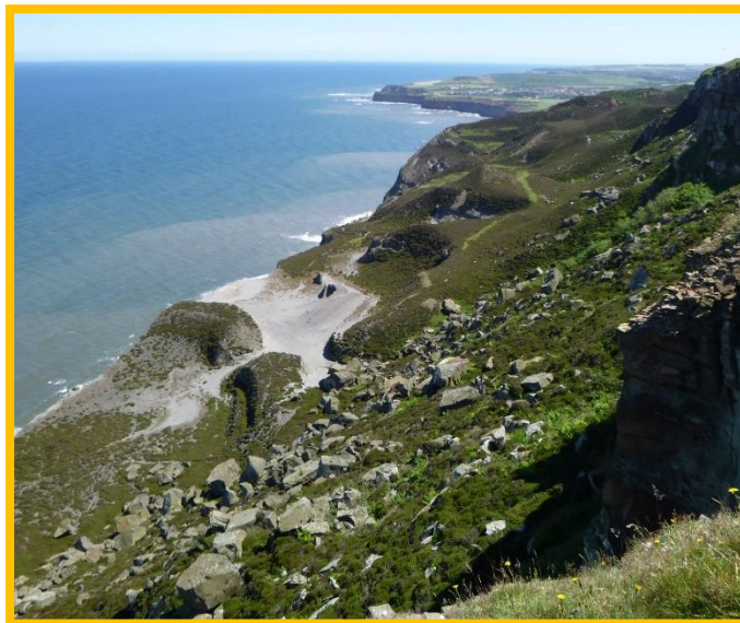
E58/5 to E58/2 – Cliffs of the Loftus Alum Quarries (Locally Active upper sections and Partly Active lower sections)
