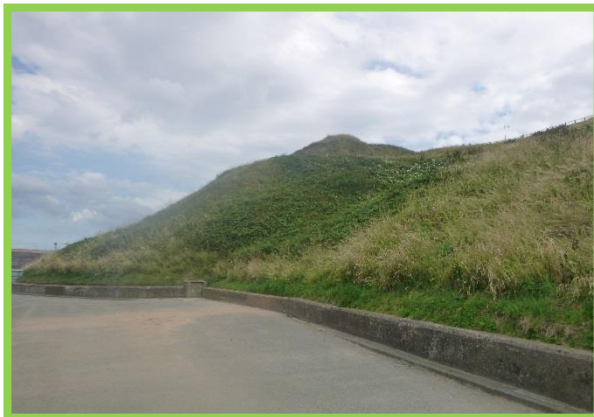
View looking east (E52/3b)
