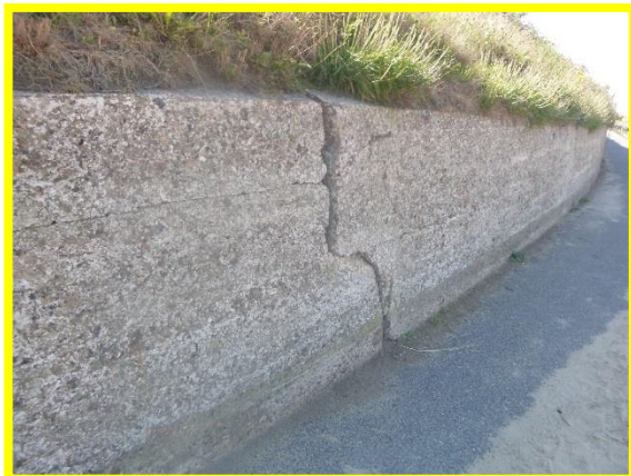
Crack in wall – no apparent change (/C0702C03)
