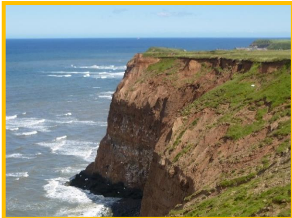
E58/1 to E59/6 Soft, slumping, upper till resting upon harder rock (Partly Active)
