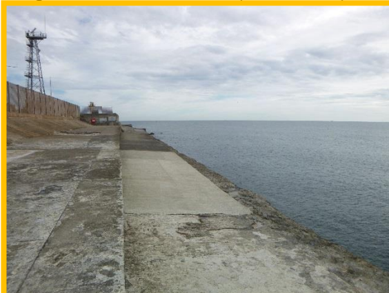
Historic repairs to deckslab along eastern face (/C0506C01)
