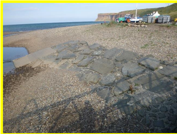
Exposed crest of grouted rock revetment (C0704C06)
