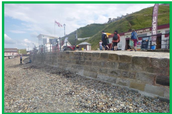
Exposed masonry at slipway (/C0702C04)
