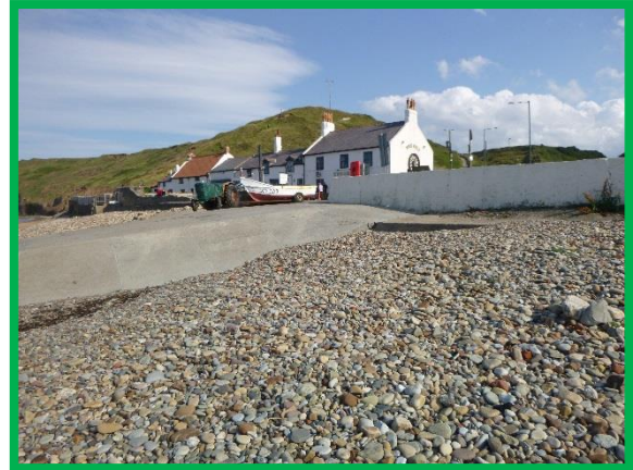
Western face of concrete slipway (/C0704C03)
