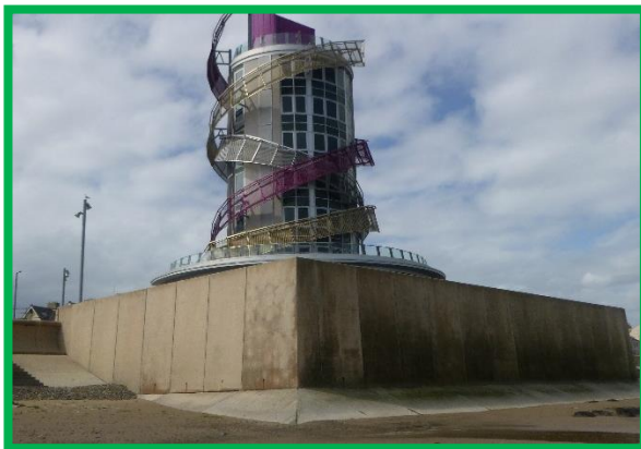
Concrete sea wall at Redcar Beacon (/C0602C03)
