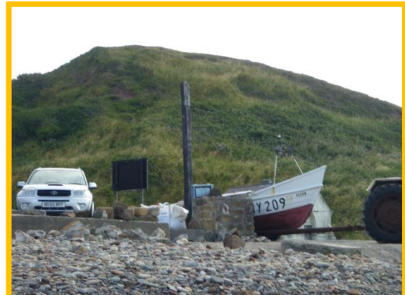
Damage to boundary wall fronting Public House (/C0704C05)
