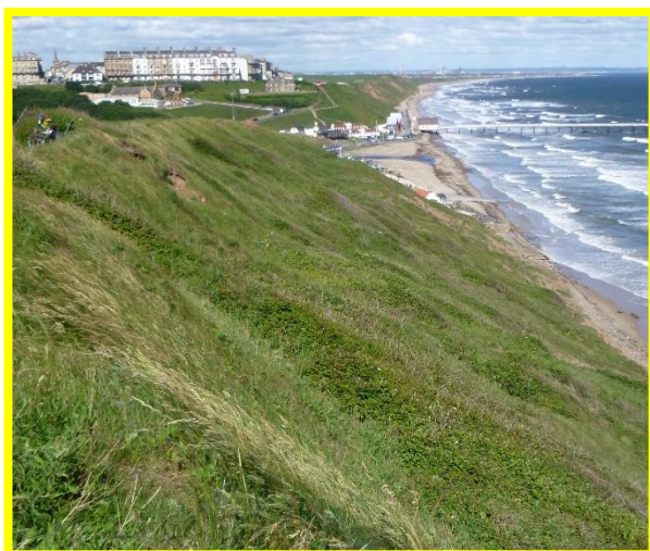
E53/3 to E53/1 Generally small-scale slumping in the till layer of the cliff northeast of Saltburn (Locally Active except E53/2, right).
